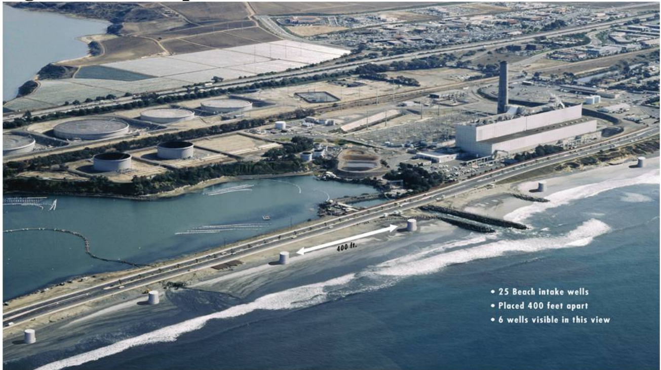
Figure 4-6 – Submerged Seabed Intake System
